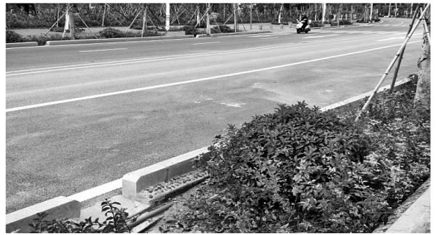
图 2 厦门市翔安新区分车绿带海绵化 Fig. 2 Spongy green belt in dividing stripes of Xiang'an New Area in Xiamen
